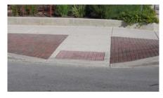
the original TAS requirements that the curb ramp have a contrasting color and textures for the entire width and depth still applies to all curb ramps in the private development. If the owner wishes to use truncated domes, they cannot extend for a depth of only 24-inches but must cover the entire length of the curb ramp.
